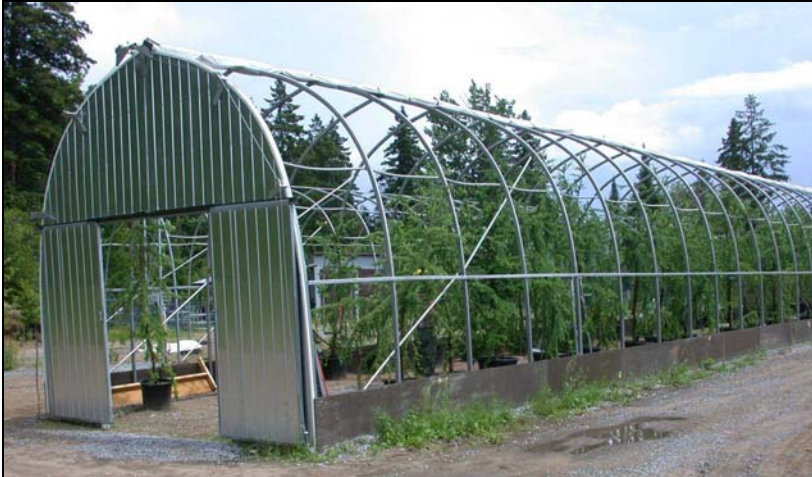
Figure 1. Shelter adapted to grow containerized larch grafts. Following pollination, tunnel covers are removed to provide optimal light conditions. (Photo: F. Colas, MRNFP)
